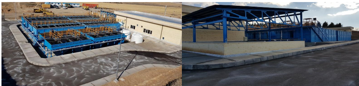
Wastewater Treatment Plant, Zanzan University Main campus
