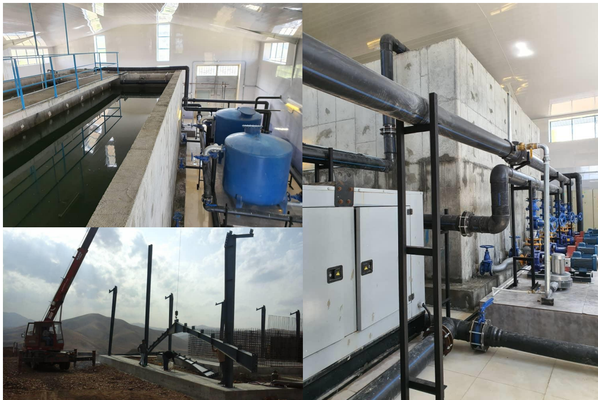
Water Treatment Plant, Qolyan-Sanandaj
