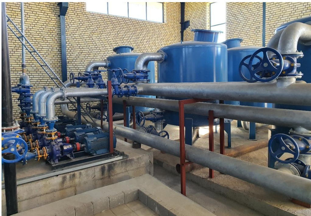
Figure ۳ Water Treatment Plant, Sarajooi-Maraqeh
