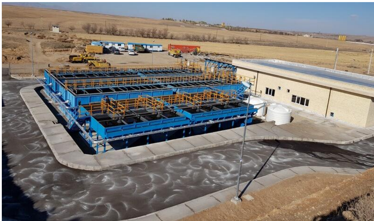
Wastewater Treatment Plant, Zanjan University 1 Figure
